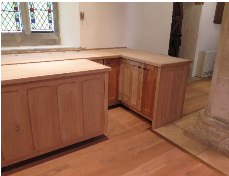
The new servery with movable section; when not in use everything is concealed below the top surfaces.
