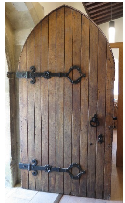
The Church Door now restored
